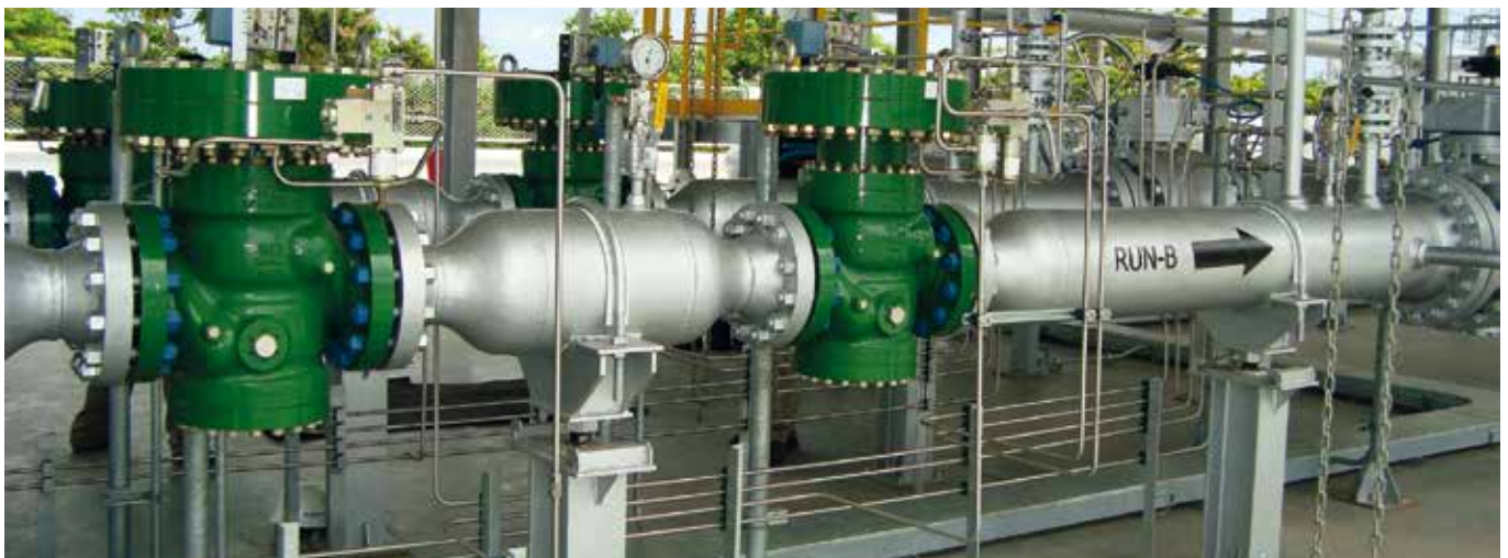
TA-956 FC and MFO DN150 ANSI 600 Customer: Ivalsa Project in Sipco Bangkok, Thailand
