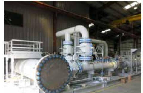
PROJECT: RLNG TERMINAL KARACHI
